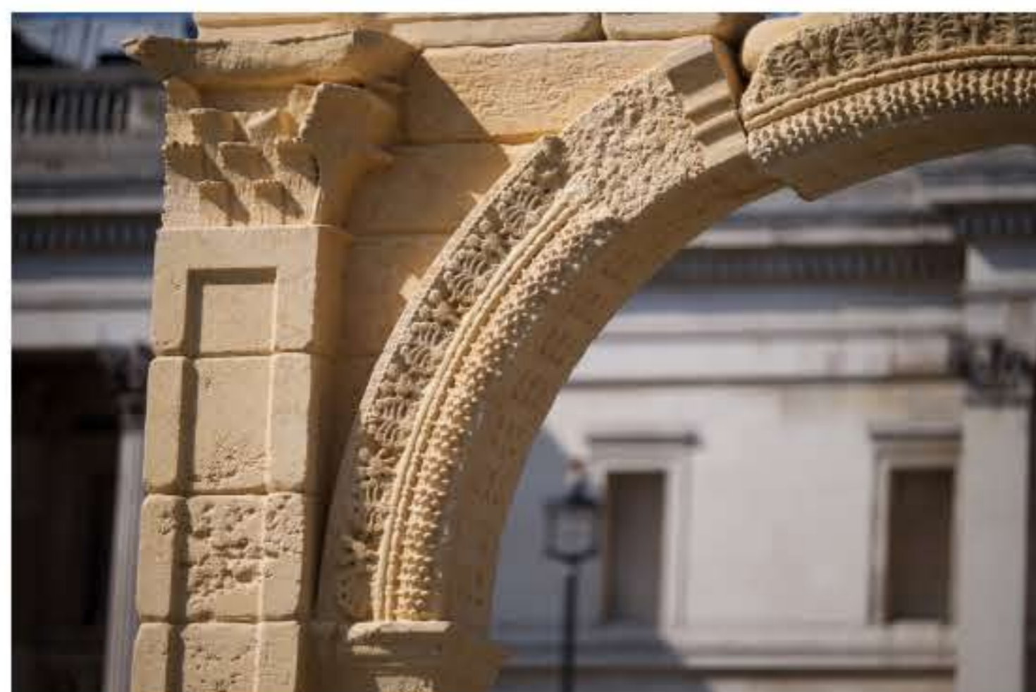
Detail on the arch was recreated using a 3D printer and data gathered from thousands of images. The reconstruction weighs nearly 11 tonnes. (Mel Hattie/CBC)
